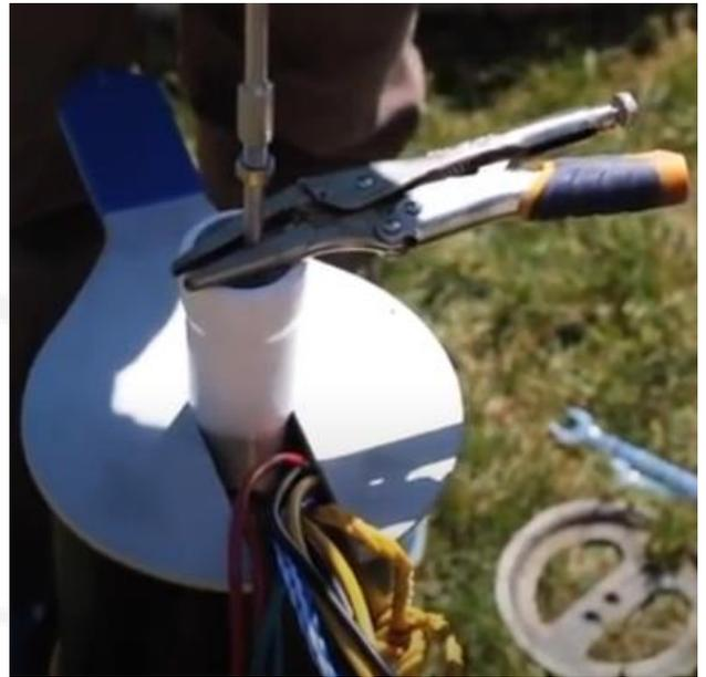
Verify that the paddle is sitting in the middle of the casing with the rope in the slot. Be careful that the rope and any wires remain in the slot through-out the installation process to prevent cutting of the rope or wires by the paddle.
