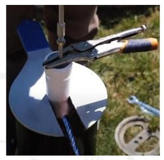
Verify that the paddle is sitting in the middle of the casing with the rope in the slot. Be careful that the rope remains in the slot through-out the installation process to prevent cutting of the rope by the paddle.
