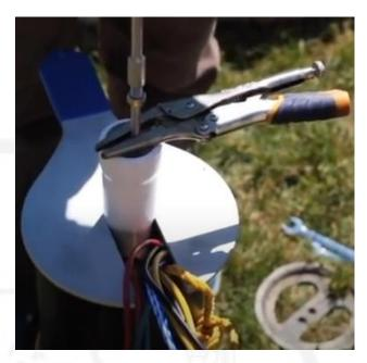
Verify that the paddle is sitting in the middle of the pump support stand with the rope in the slot. Be careful that the rope and any wires remain in the slot through-out the installation process to prevent cutting of the rope or wires by the paddle.
